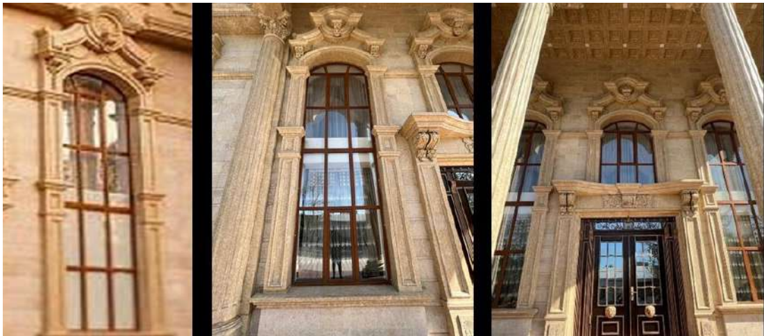
Figure 23. Window and door of the wedding hall
